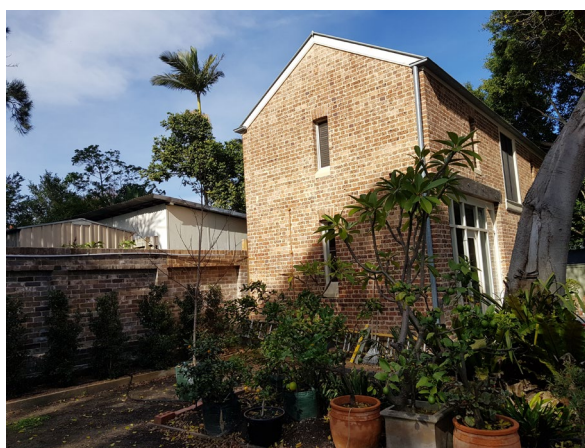
Image E. Existing rear dwelling, former stable
